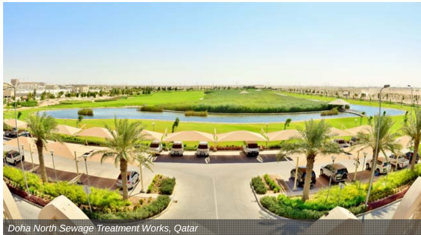
Doha North Sewage Treatment Works, Qatar
