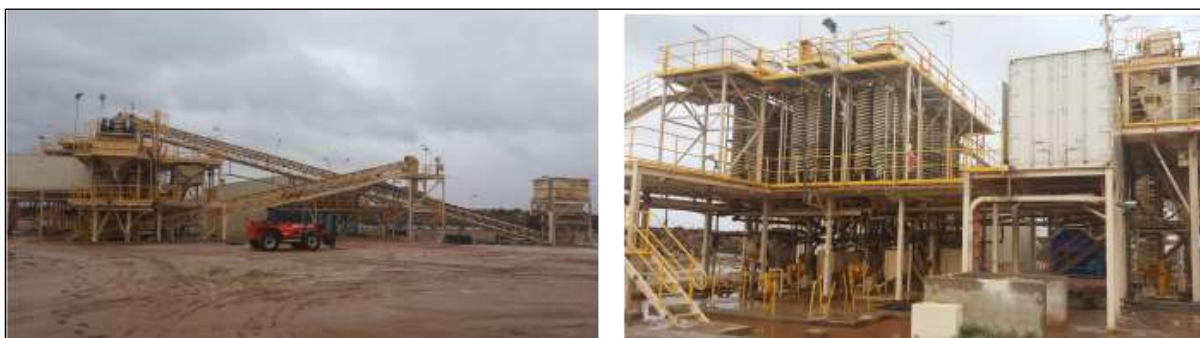
Figure 21: Photos of processing plant at Bald Hill.
