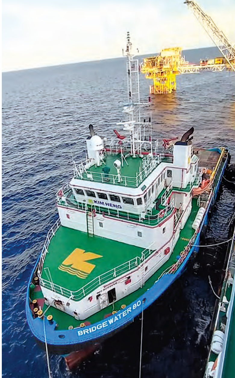
Offshore Platform Works
