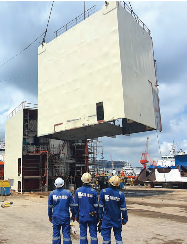
Scrubber Fabrication (External)
