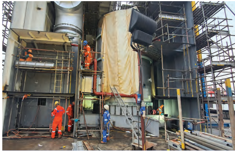
Scrubber Fabrication (Internal)
