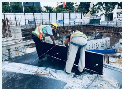
Workers using SRL when working near unprotected edge.
