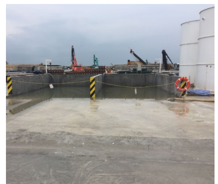
New water tanks and ground pits for collection of rainwater.
