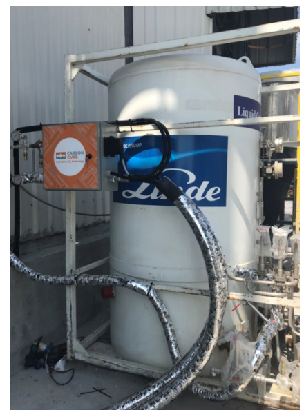
CarbonCure system at a PanU plant.
