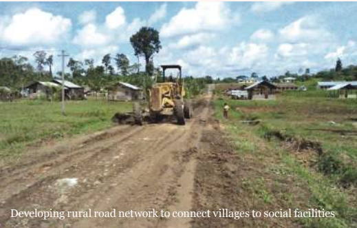
Developing rural road network to connect villages to social facilities
