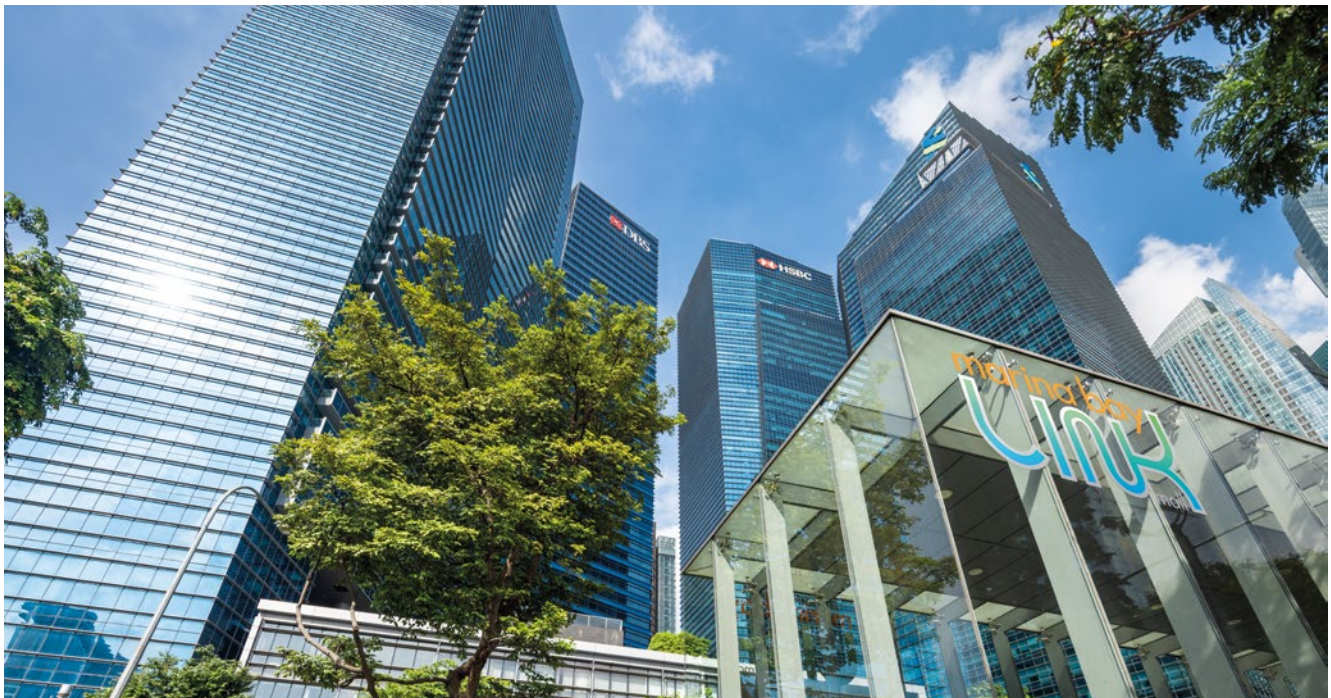
Keppel REIT's sterling portfolio of properties includes Marina Bay Financial Centre in Singapore, an integrated development comprising three premium Grade A office towers and the subterranean Marina Bay Link Mall.
