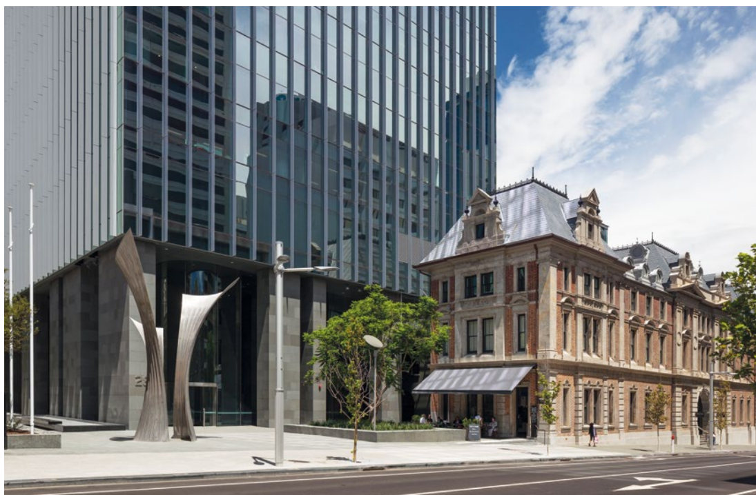
David Malcolm Justice Centre is located in Perth's CBD and has the Minister for Works – Government of Western Australia as its principal tenant.
