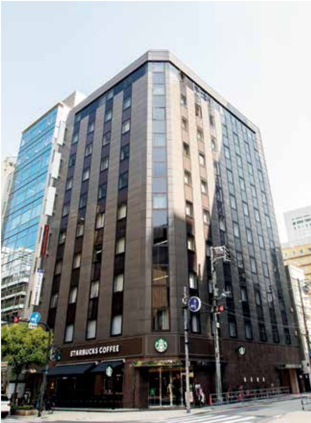
YOTSUBASHI EAST BUILDING AT THE CORNER OF YOTUSBASHI SUJI, SHINSAIBASHI • LAND AREA - 525 SQM • GFA - 4,695 SQM • EFFECTIVE OWNERSHIP - 50%
