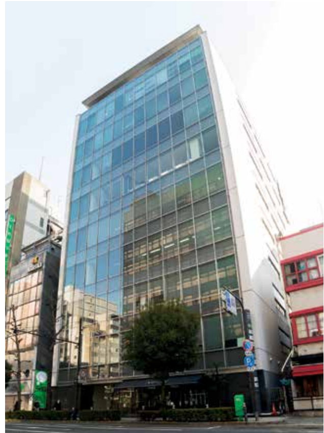
YOTSUBASHI NAKANO BUILDING ALONG YOTUSBASHI SUJI, SHINSAIBASHI • LAND AREA - 806 SQM • GFA - 7,925 SQM • EFFECTIVE OWNERSHIP - 50%
