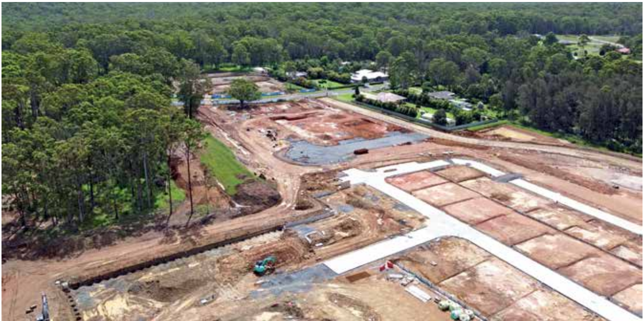
CONSTRUCTION COMMENCED IN Q3 2021 AND IS WELL UNDERWAY
