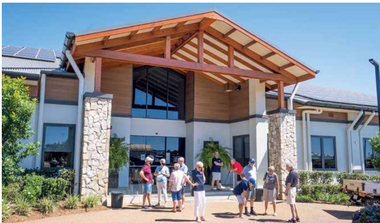
HIGHFIELDS COUNTRY LIVING OPEN DAY HELD IN OCTOBER 2021. CONSTRUCTION OF STAGES THREE AND FOUR HOMES WELL UNDERWAY, STAGE FIVE PROGRESSING WELL WITH CIVILS WORKS COMPLETED IN Q1 2022
