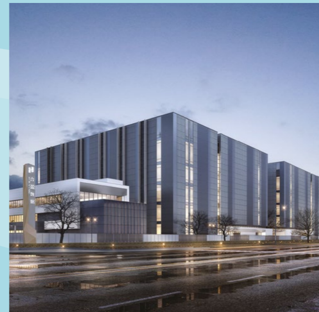
Data centre in Greater Beijing, China
