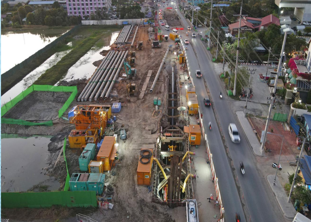
Direct Pipe construction works in Bangkok, Thailand
