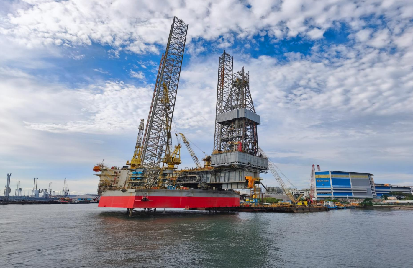
Providing loading, scaffolding, offloading, and piping services for a jack-up rig at Penjurong Yard
