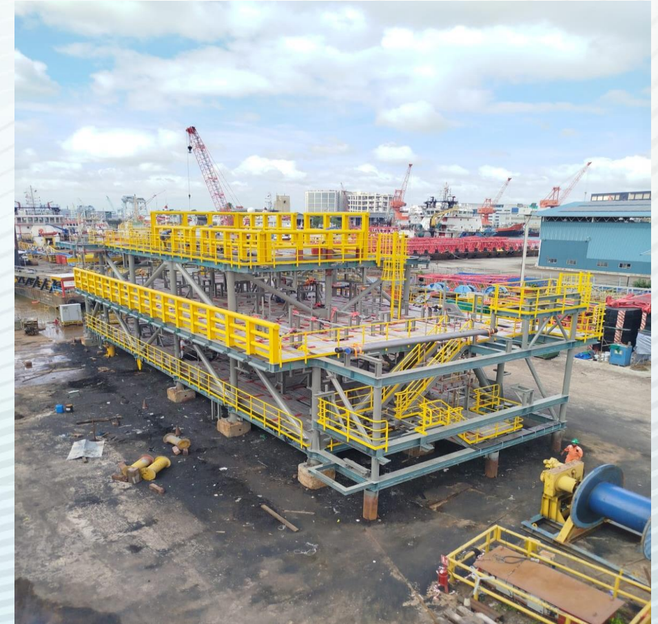
Fabrication and assembly of Jaguar module
