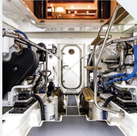
STRATEGIC CARBON-FIBER CONSTRUCTION
