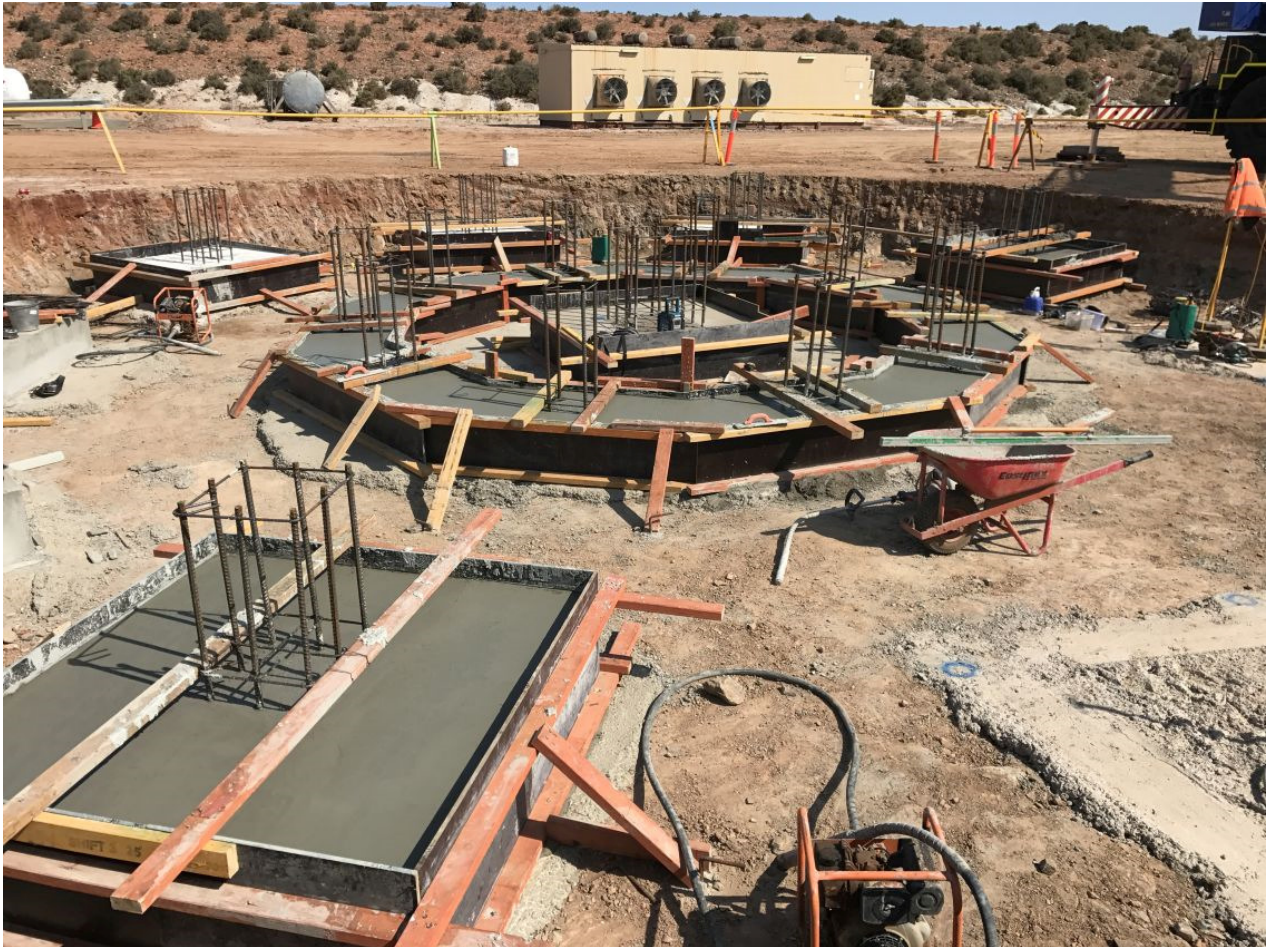
Figure 4 | Concrete works for Thickener
