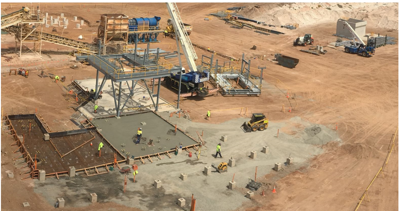
Figure 5 | Feed Bin Wall & Concrete Footings completed
