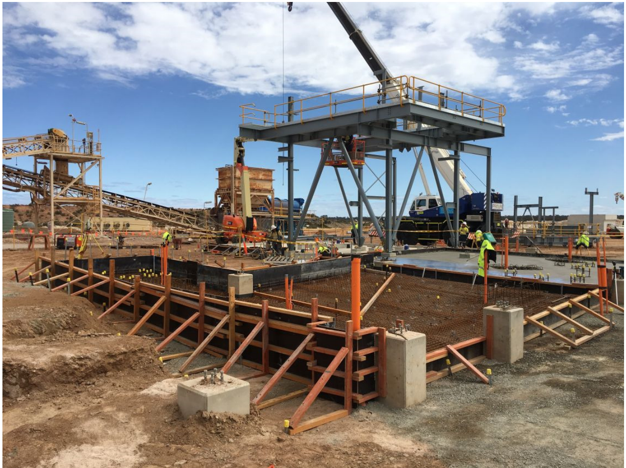
Figure 6 | Structural Steelwork being erected
