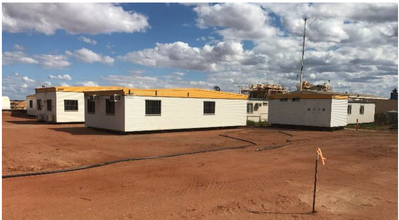
Figure 7 | New site offices in position
