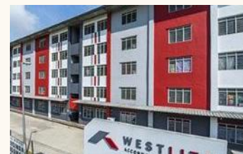
Westlite Senai, Johor Malaysia – assessment in progress
