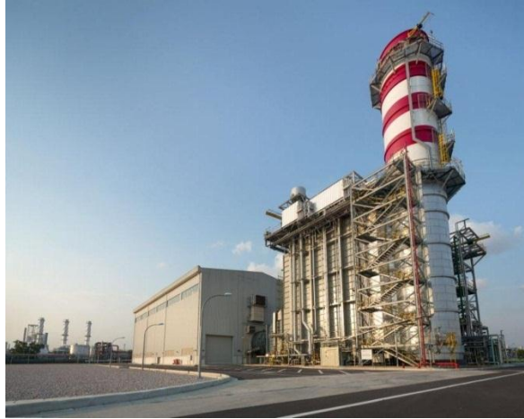
Sembcorp's new cogeneration plant located in the Banyan area of Jurong Island.
