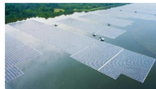
60 MWp system at Tengeh Reservoir
