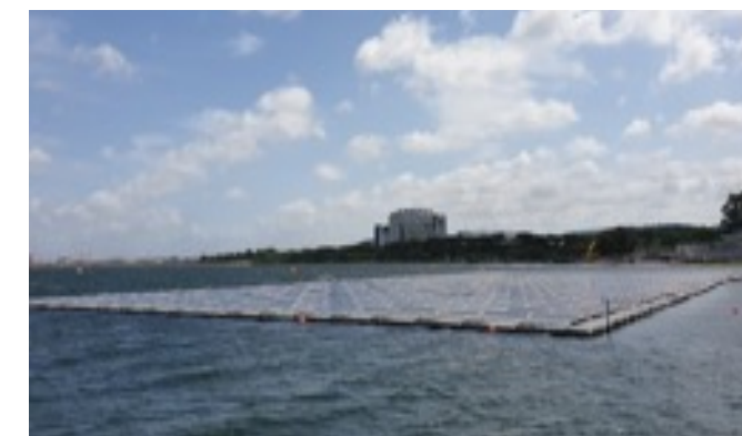
1.5 MWp system at Lower Seletar Reservoir
