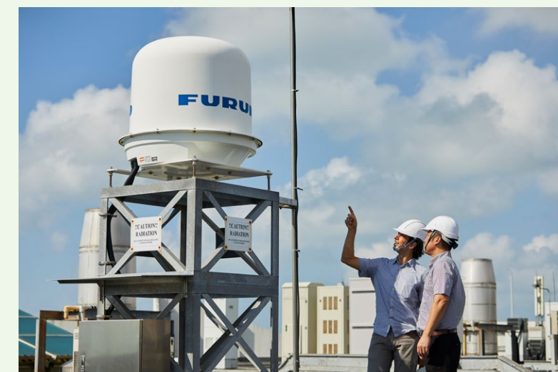
Radar at Changi Water Reclamation Plant
