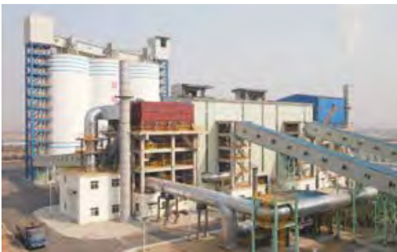
Qingdao JV plant
