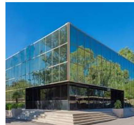
2601 West Broadway Road, Tempe
