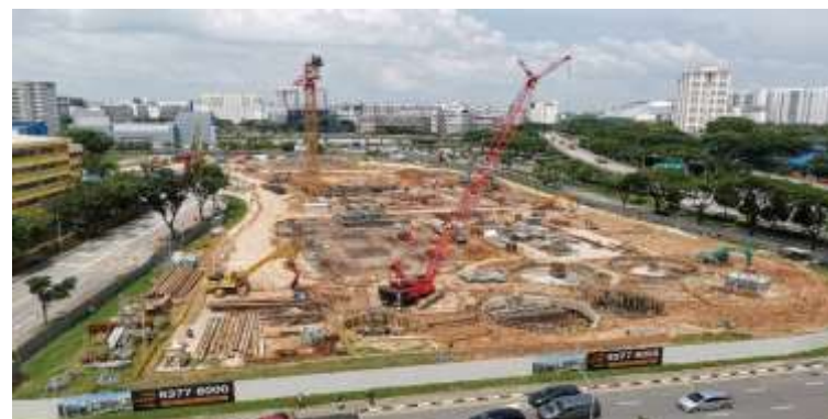
Completed piling for Block 1 and 2. Substructure works in progress
