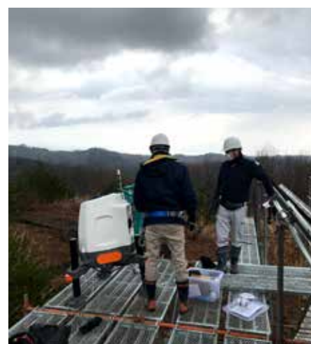
LiDAR set up in process
