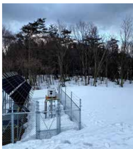
Powering of LiDAR equipment using only PV panels
