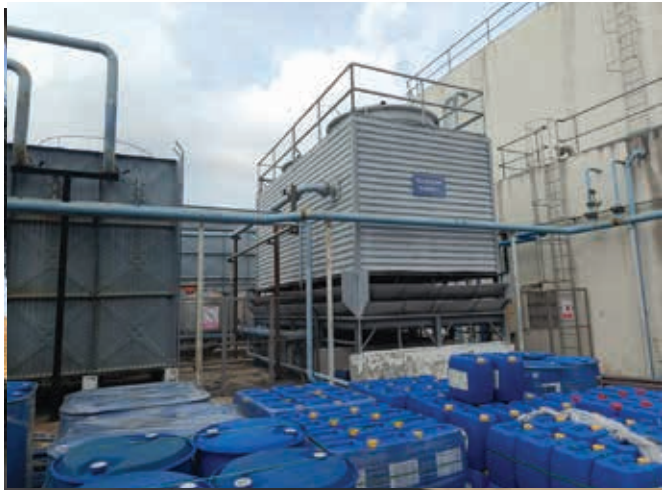
Enhancement of cooling tower system
