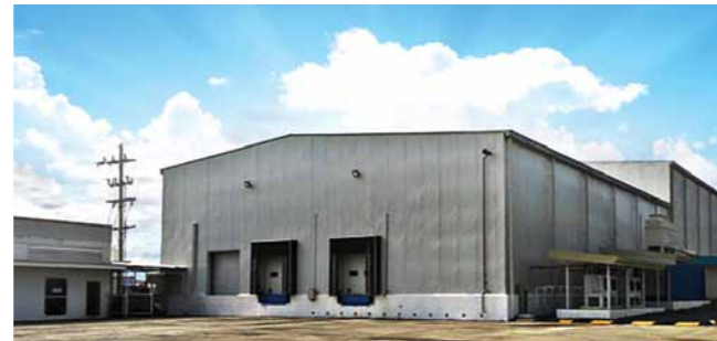
Del Monte's new processing facility in the Philippines that produces frozen pineapple
