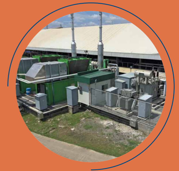
The generator sets for the waste-to-energy facility
