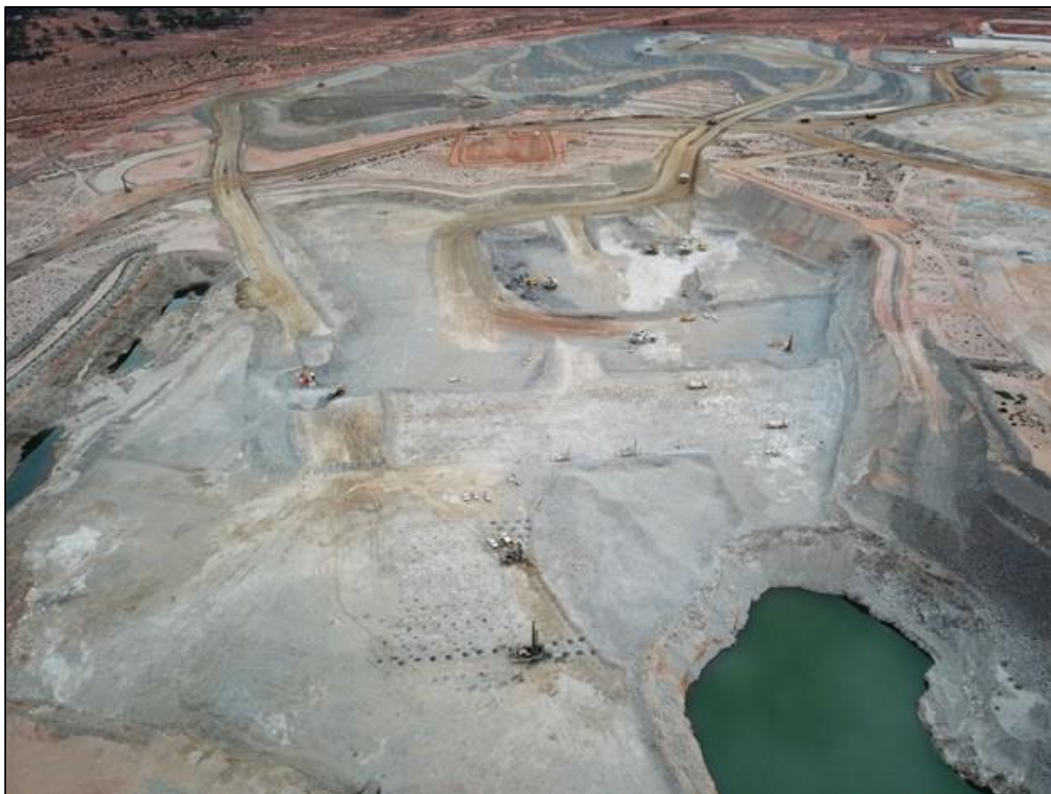
Figure 37: Current Stage 1 pit
