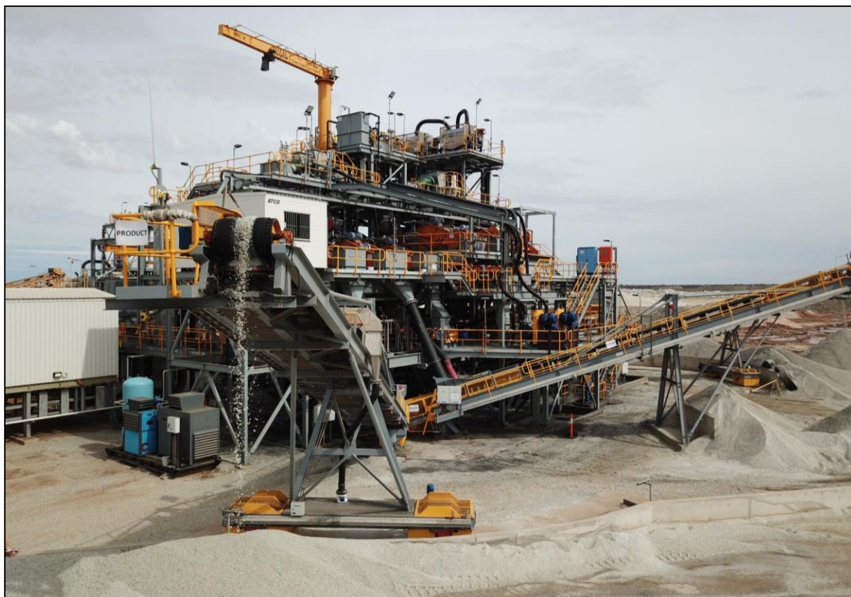
Figure 20: Stage 1 DMS plant
