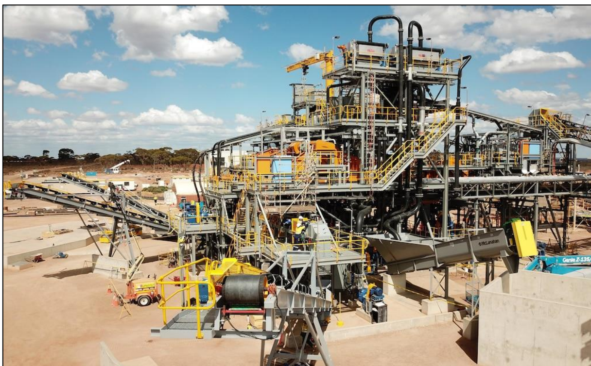
Figure 19: The Bald Hill media separation plant
