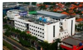
Siloam Hospitals Kebon Jeruk
