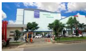
Siloam Hospitals Purwakarta
