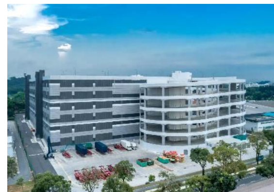
20 Tuas Avenue 1, Singapore
