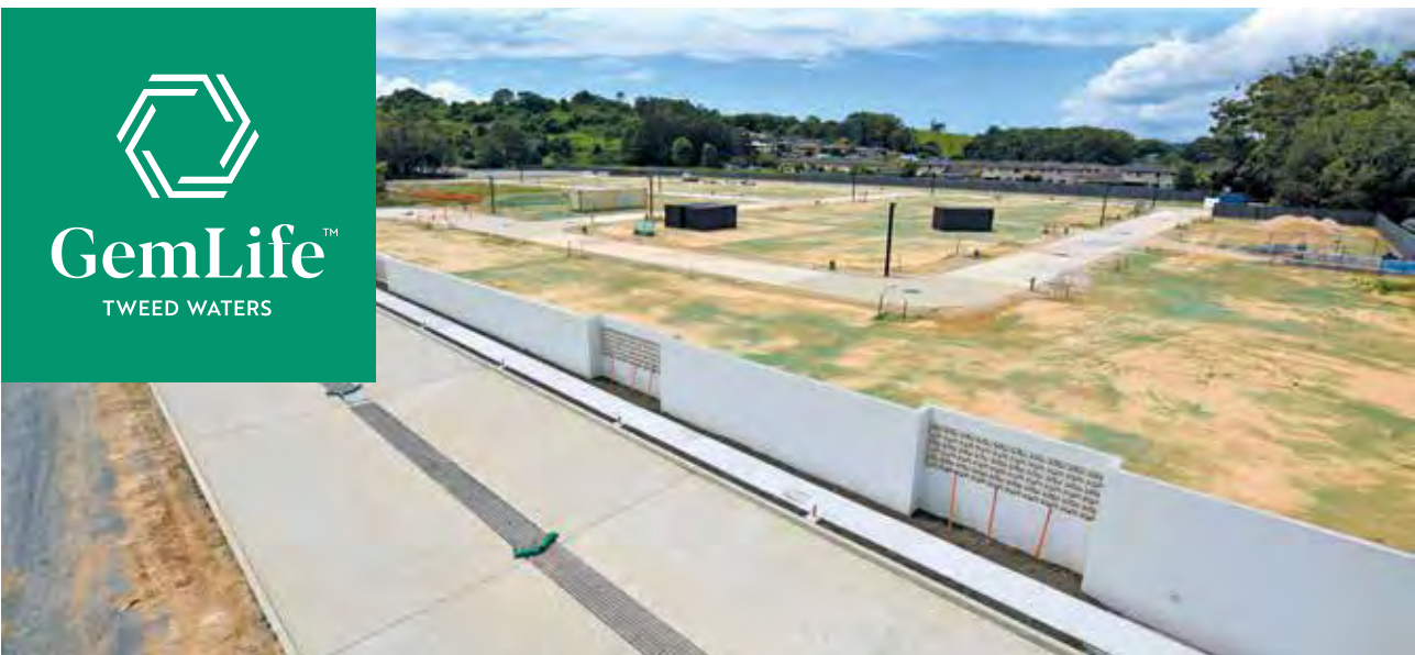
BULK EARTHWORKS AND CIVIL WORKS FULLY COMPLETED IN NOVEMBER 2022
