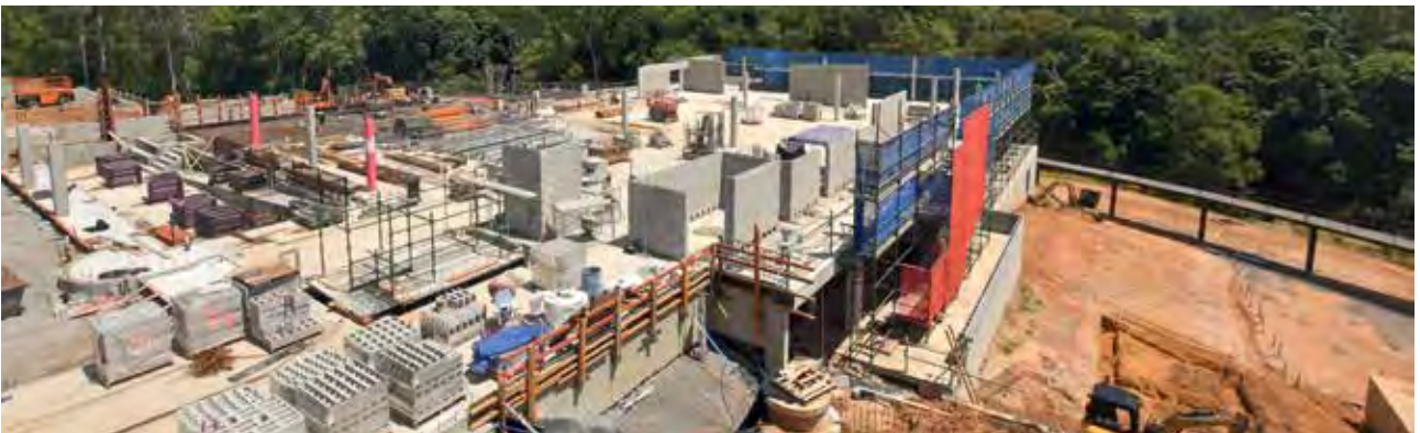
CONSTRUCTION FOR COUNTRY CLUB COMMENCED IN FEBRUARY 2023
