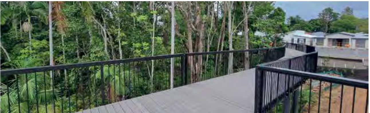
313 METRES OF ELEVATED BOARDWALK TAKING SHAPE
