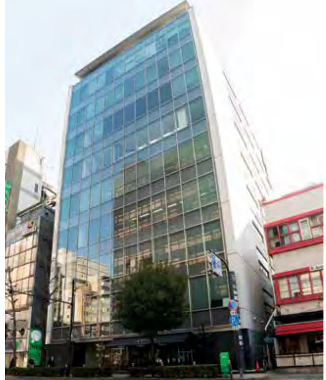
YOTSUBASHI NAKANO BUILDING ALONG YOTSUBASHI SUJI, SHINSAIBASHI • LAND AREA - 806 SQM • GFA - 7,925 SQM • EFFECTIVE OWNERSHIP - 50%
