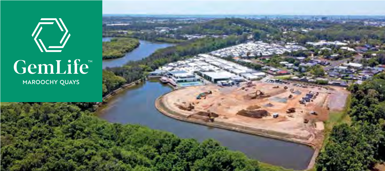
CONSTRUCTION FOR AN OFF-SITE CARAVAN STORAGE COMPOUND IN KULUIN AND STAGE FOUR OF THE RESORT COMMENCED IN Q3 AND Q4 2022 RESPECTIVELY
