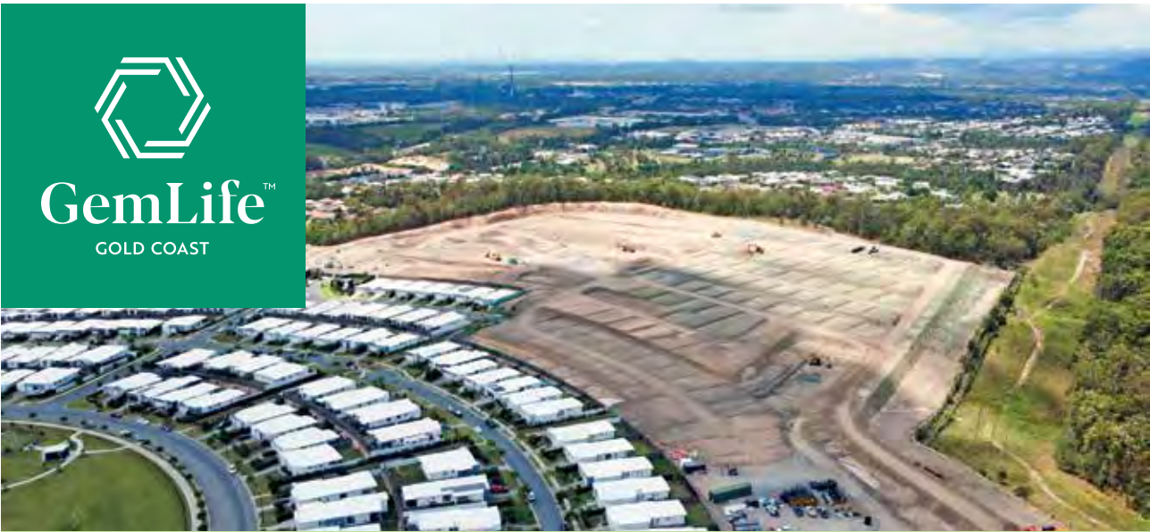
BULK EARTHWORKS IN STAGES TWO AND THREE ARE MOVING AHEAD
