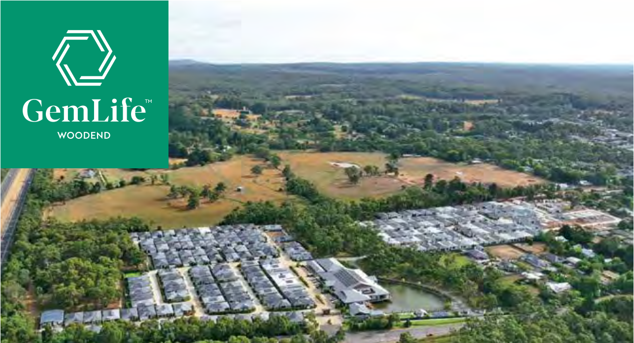
FINAL STAGE OF RESIDENTIAL HOMES CONSTRUCTION COMMENCED IN NOVEMBER 2022
