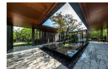
Yanlord Four Seasons New Gardens, Shenzhen 仁恒四季新园, 深圳
