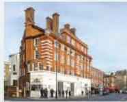
Former Westminster Fire Station, United Kingdom
