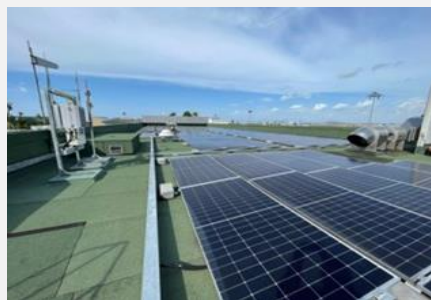
Solar panel installation at 50 Airport Boulevard, Singapore
