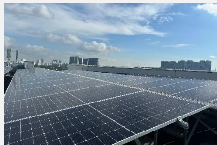
Solar panel installation at 4 Tuas Avenue 5, Singapore
