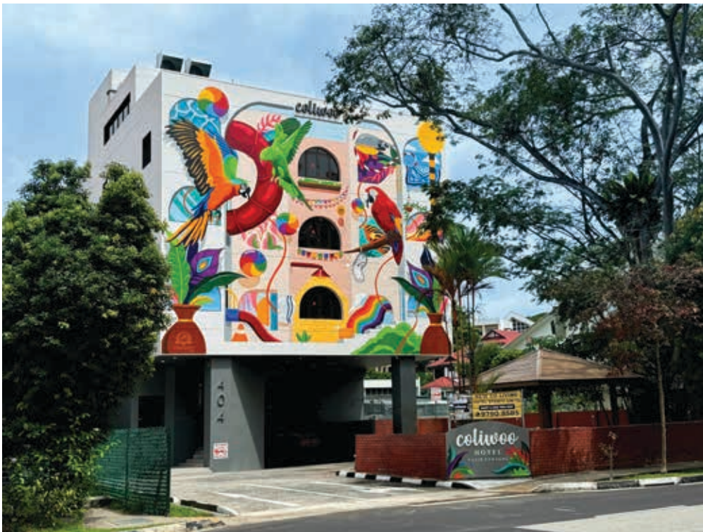
Exterior of Coliwoo Hotel Pasir Panjang, featuring an imaginative mural that injects vibrancy within the neighbourhood of the Pasir Panjang district
