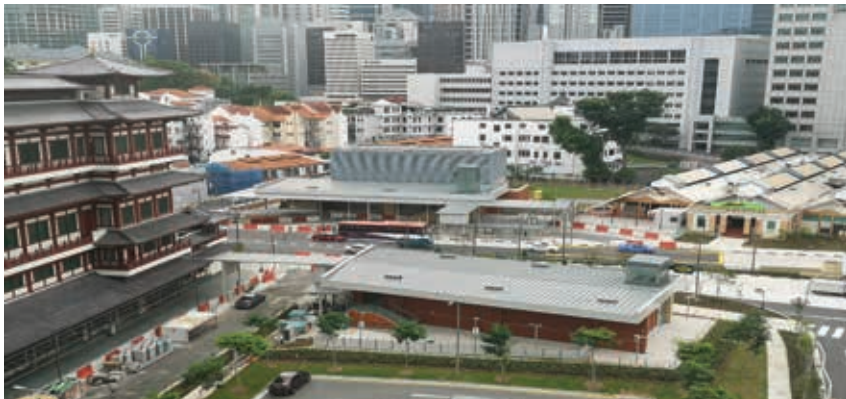
Maxwell Station for Thomson-East Coast Line substantially completed in October 2021
