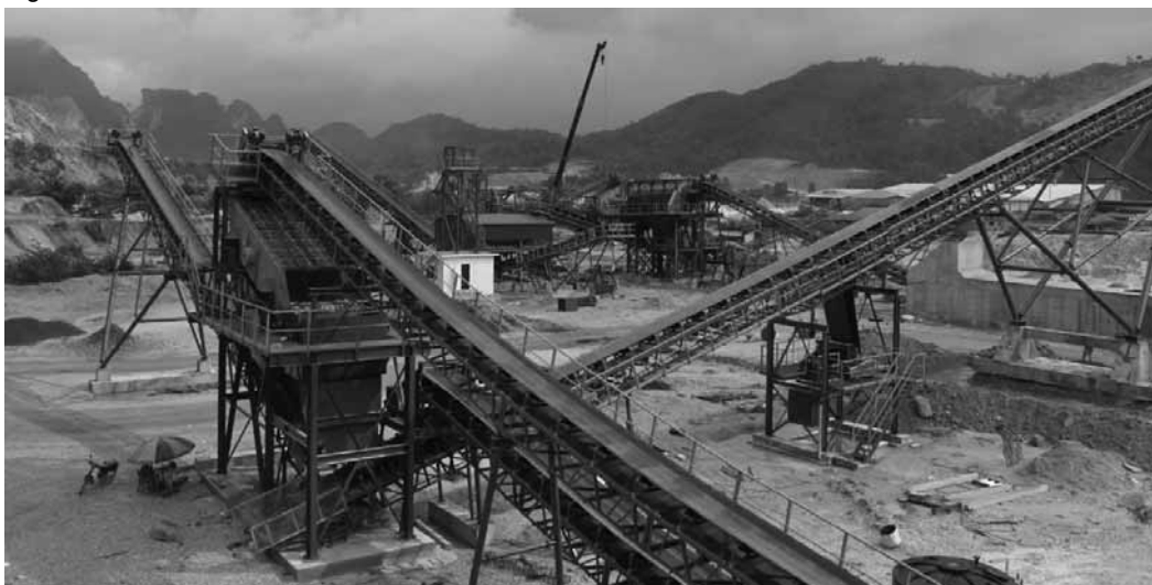
Figure II - 6 Crusher Installation at HAM Mine
