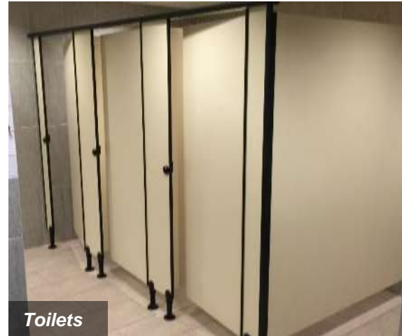
Upgrading at PSA Building (before)
