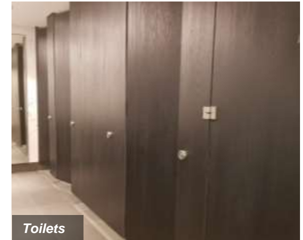
Upgrading at PSA Building (after)
