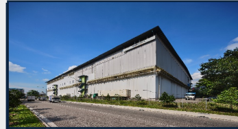
2 ALOG Cold Centre 2 Fishery Port Road
