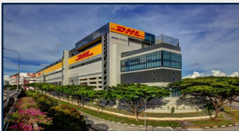
10 DHL Supply Chain ARC 1 Greenwich Drive
