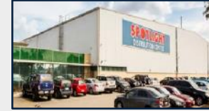
19 217 – 225 Boundary Road, Laverton North
