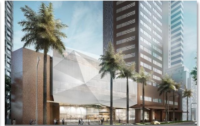
New façade facing Raffles Place Green
