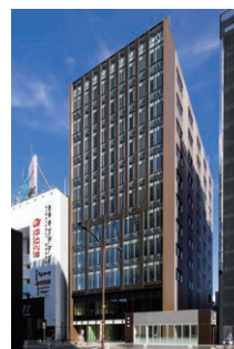
Kichijoji Fukoku Seimei Building Completion in fiscal 2023
