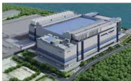
Advanced Packaging Facility
