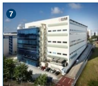
Hi-Speed Logistics Centre
