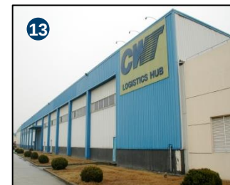
Jinshan Chemical Warehouse
