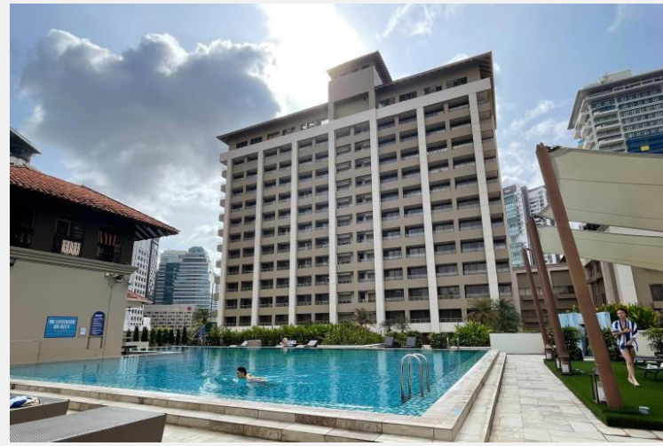
Removal of Existing Planter Boxes
