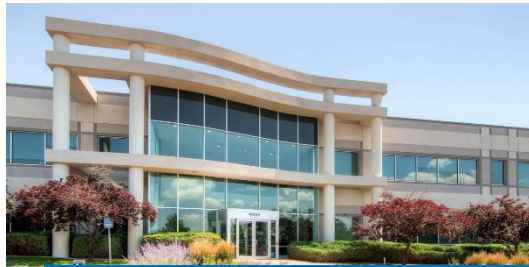
Westmoor Center, Denver
