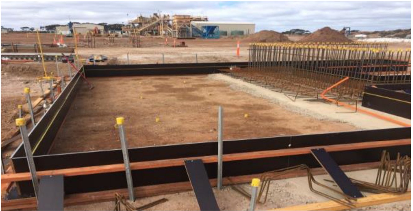
Picture 1 | Feed bin slab north end ready for blinding
