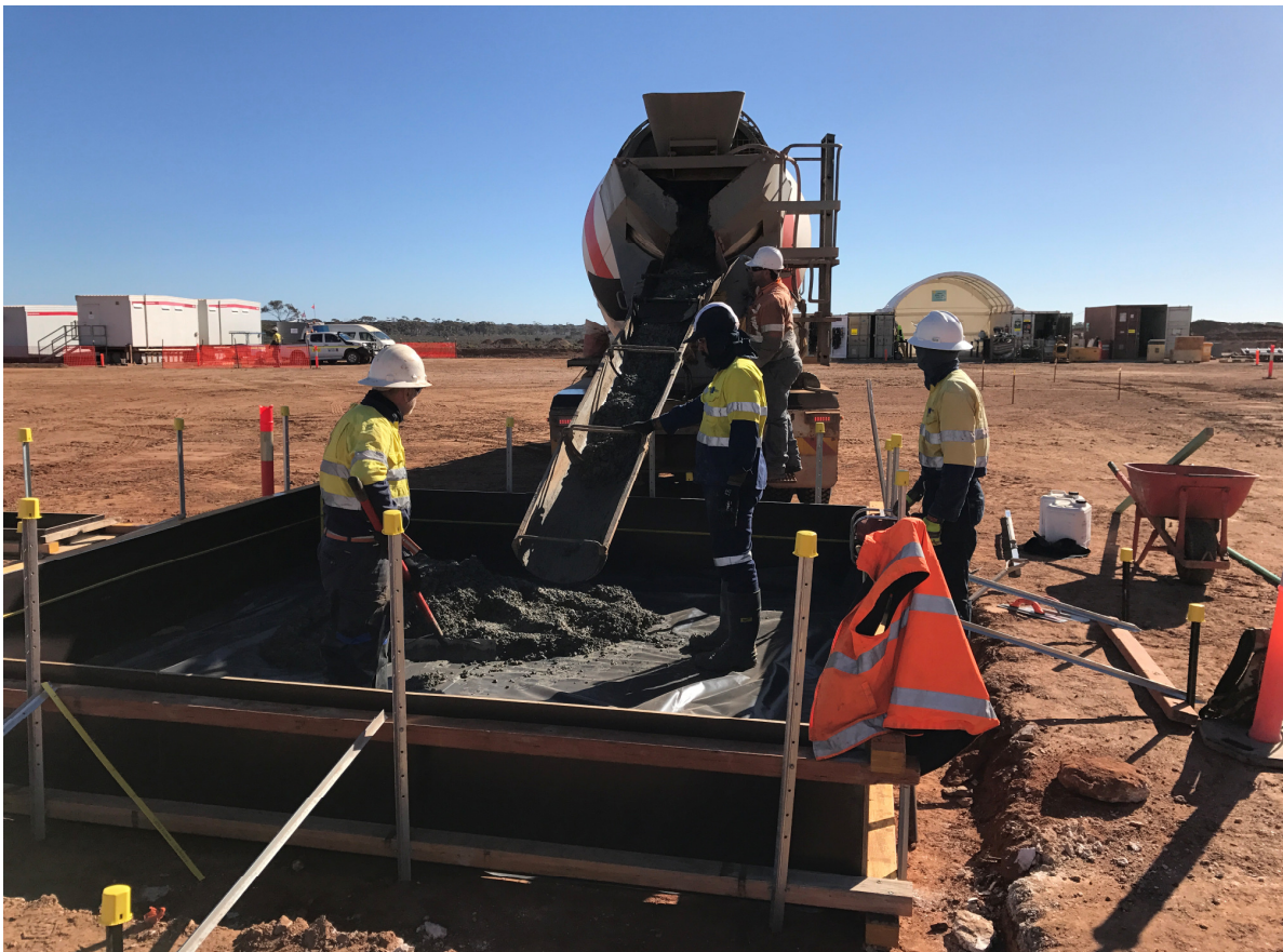
Figure 4 | First concrete pour - Take up tower curing
