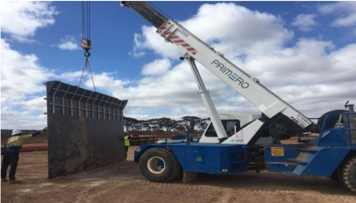
Picture 3 | Continue with cast in bar & shutter fabrication
