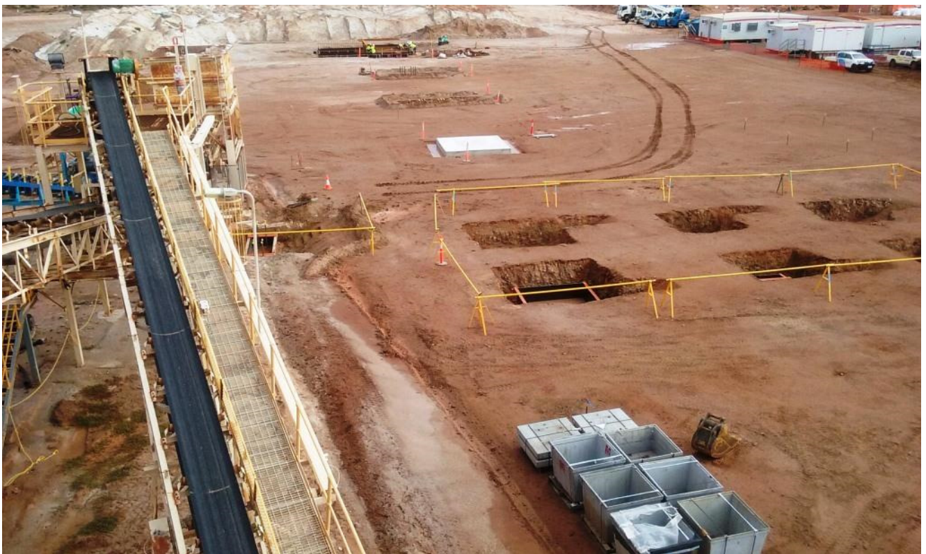
Picture 2 | Excavations for foundations
