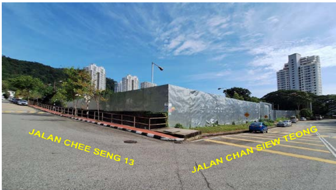
General View of Subject Property
