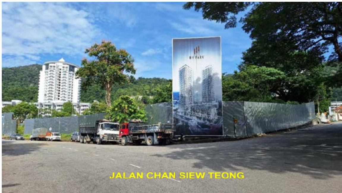
General View of Subject Property
