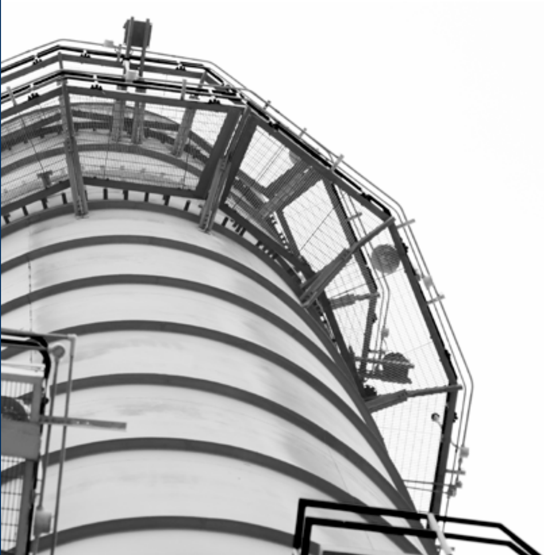
Mexicali Gas Generation
