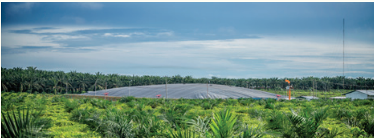
Canvas-covered methane capture lagoon in PT Tania Selatan in Sumatra, Indonesia.
