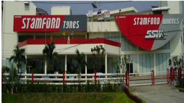
SSW wheels manufacturing factory, Nonthaburi
