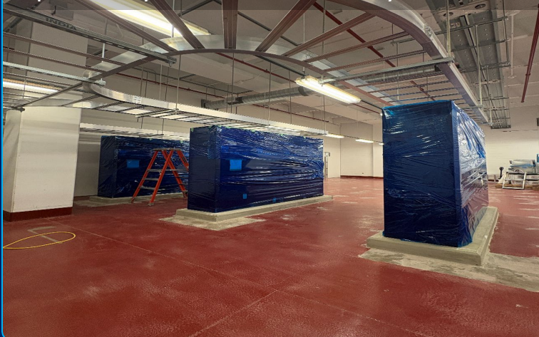
Replaced Battery Room Cabinets and Cable Tray
