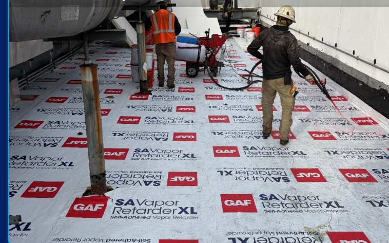
Sealed Exterior Vapor Barrier
