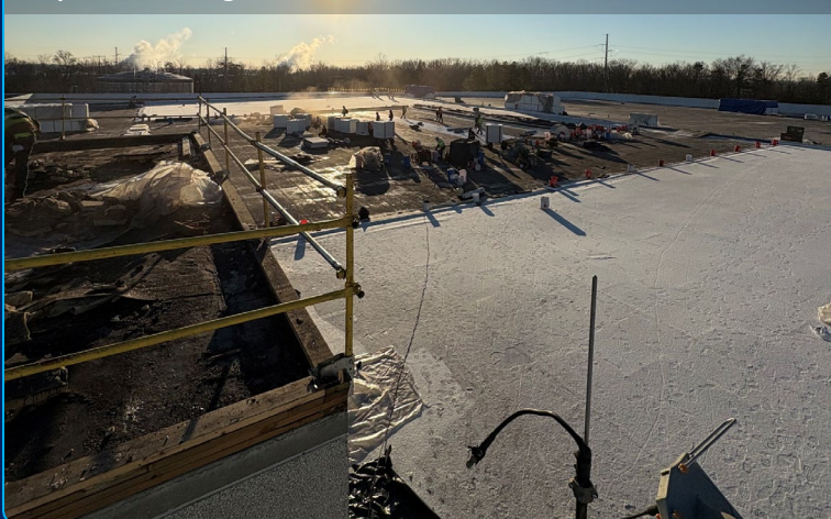
Replaced Existing Roof
