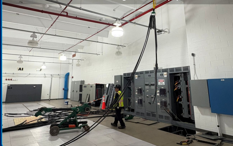
Demolished and Removed Existing Electrical Equipment
