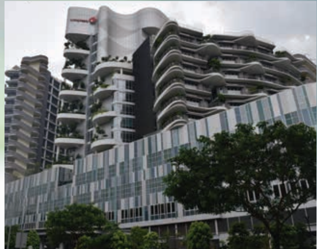
Ng Teng Fong General Hospital – valve
