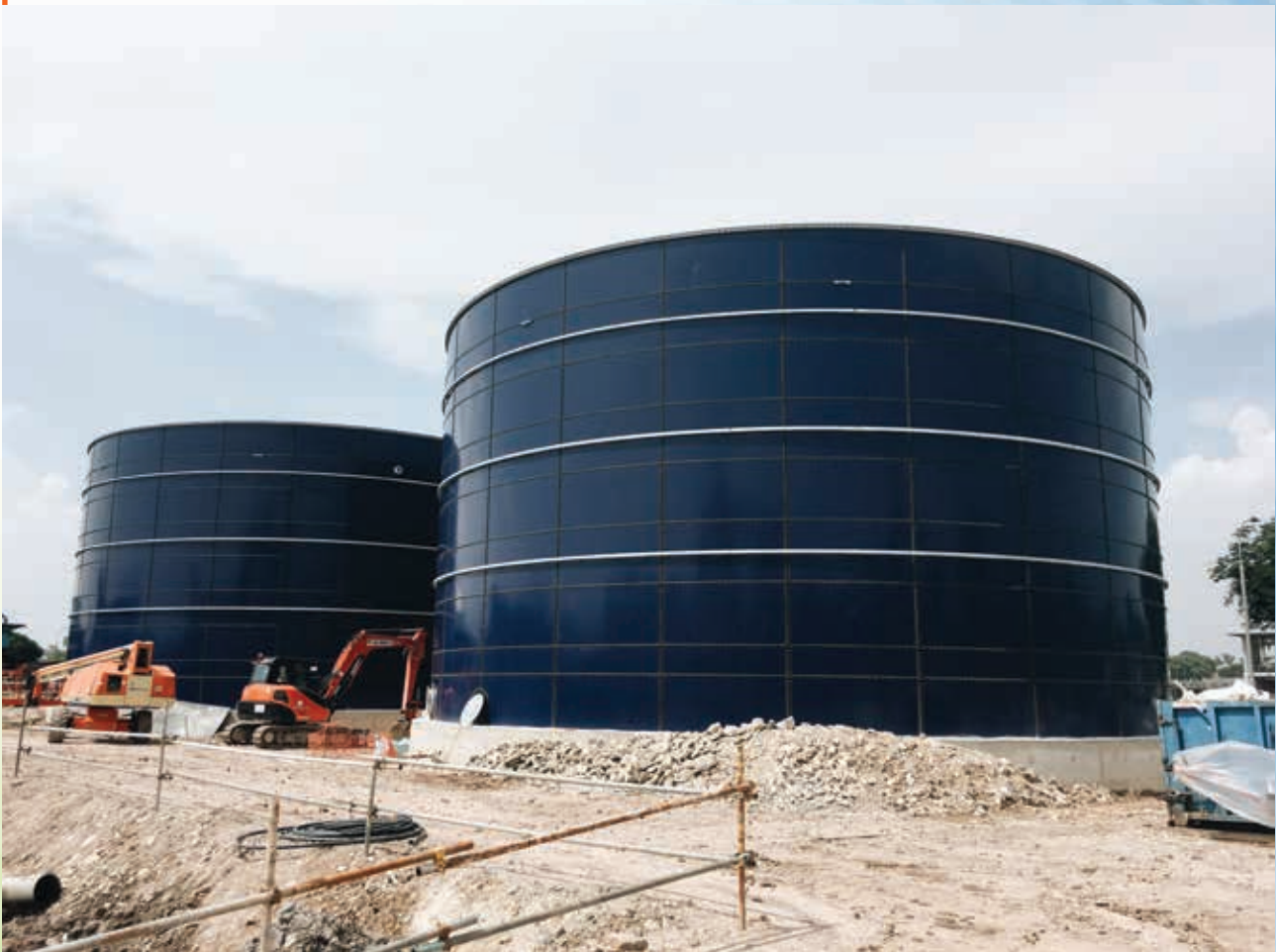
JURONG WATER RECLAMATION PLANT – bolted steel tank
