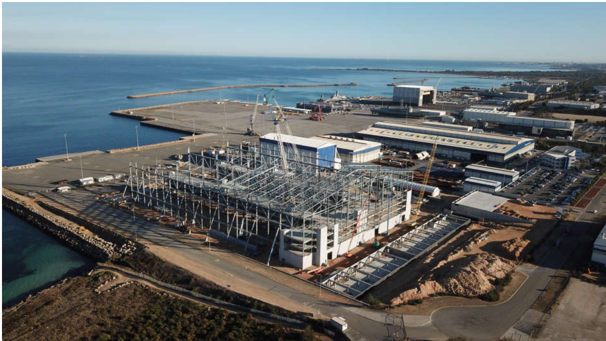
Construction of new shipbuilding and maintenance facilities at Henderson, WA, is well underway
