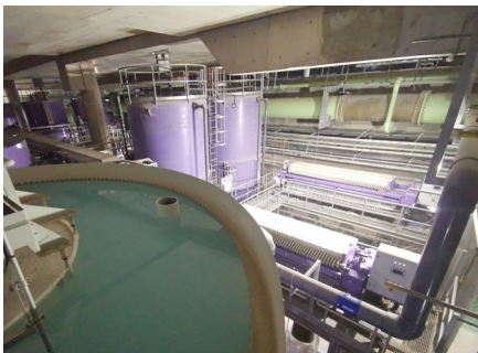
Design, manufacture, delivery, installation, training and testing & commissioning of hydrated lime storage, feed and saturation system.
