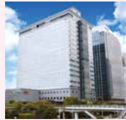
Fujitsu Makuhari Building
