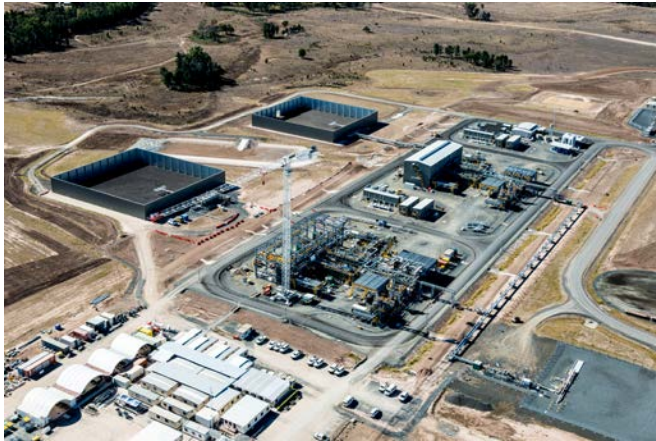
Orana Gas Processing Facility, July 2014
