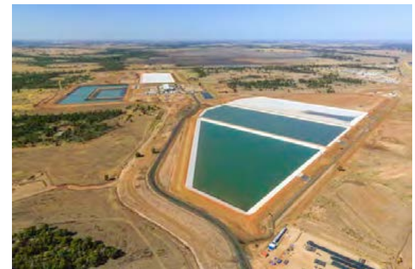
Condabri Central water and brine ponds
