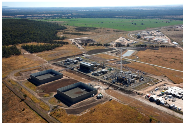
Reedy Creek Gas Processing Facility
