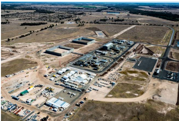
Condabri North Gas Processing Facility
