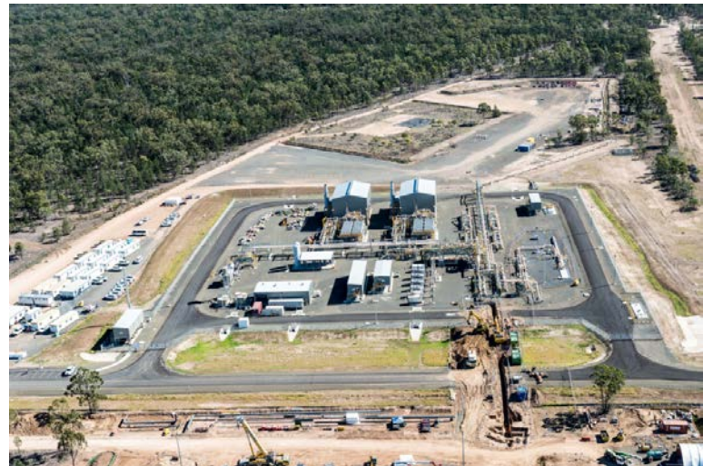
Talinga Pipeline Compression Facility, July 2014
