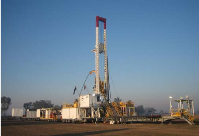
Coil-tubing drill rig
