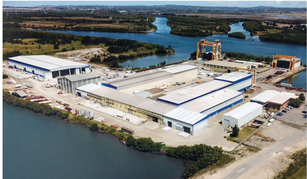
Newcastle Facility, NSW
