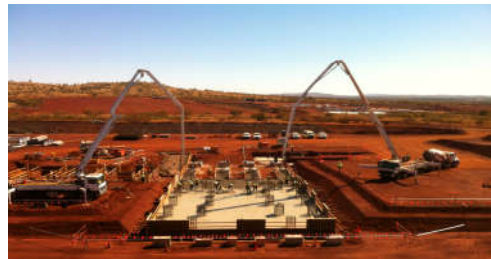
Site Civil Works
